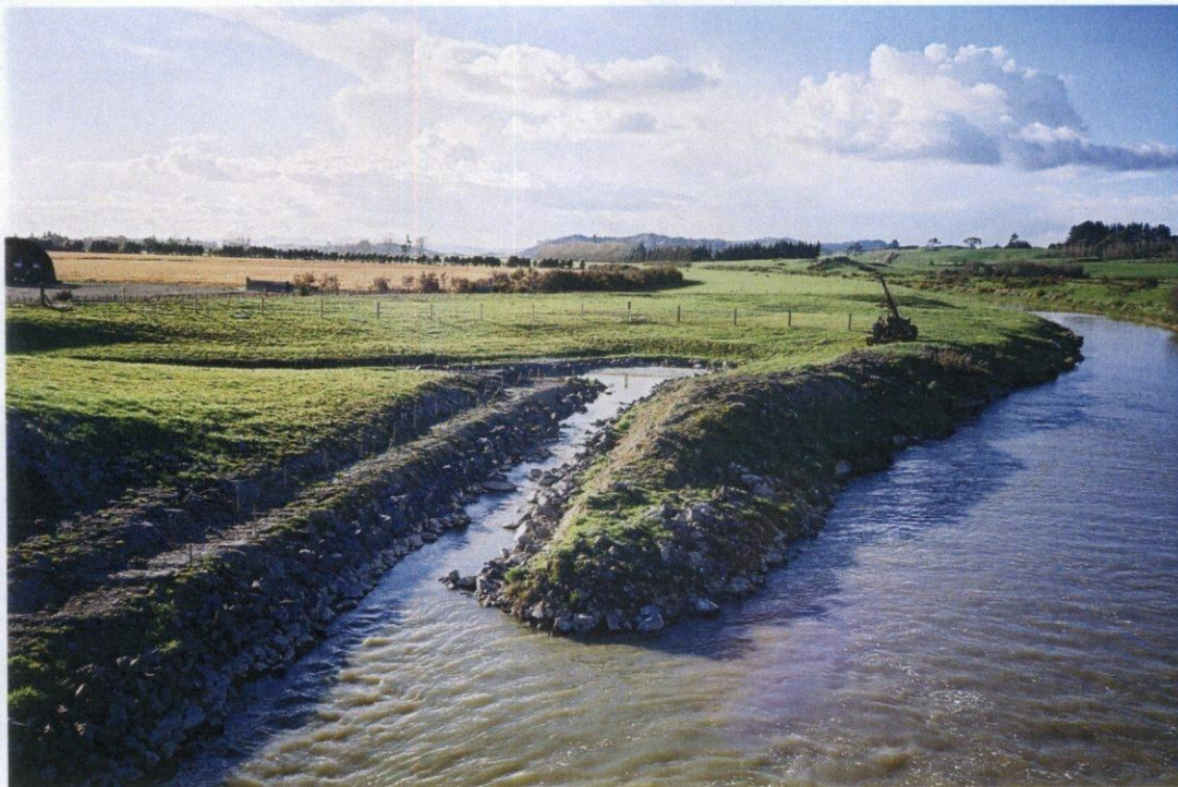
Plate 1. Lake Waikare “nature like” fish pass (on left) looking downstream from the control structure.
