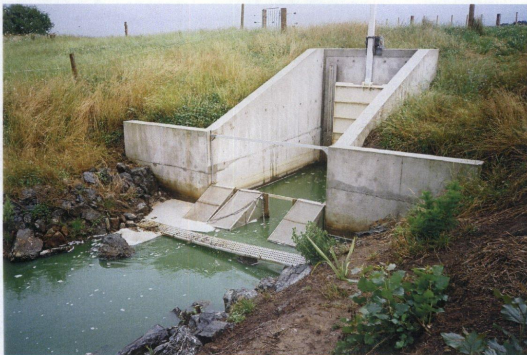
Plate 2. Lake Waikare fish pass water level control structure where the channel crosses the stop bank. Note fine mesh traps used for monitoring fish migration.
